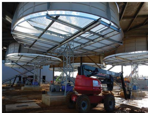
Air Cooling Condenser at the Snetterton REP, UK
