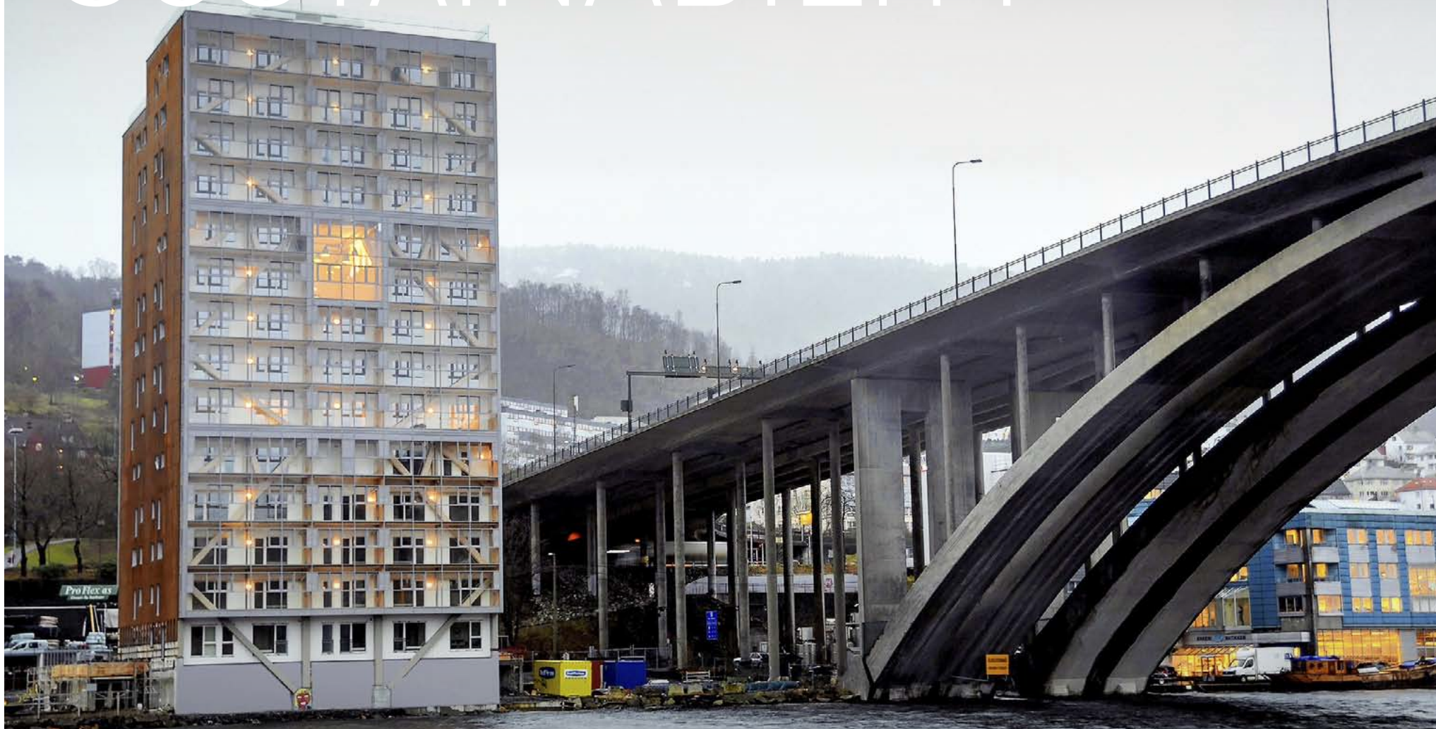
The world's tallest wooden house "Treet" in Bergen, Norway with ROCKWOOL facade insulation contributing to the apartments being built according to passive house requirements.
