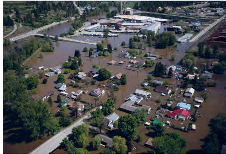
→ Flooding hits Grand Forks, British Columbia and the local ROCKWOOL manufacturing site.
