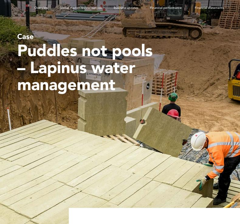
The largest ever stone wool-based water management solution, installed in Schimmert, The Netherlands, helps solve a major problem for the town: flash flooding caused by extreme rainfall. The customised solution consists of 820 m³ of Lapinus stone wool elements placed under the playground at 't Kirkeveldsje primary school. When there is heavy downpour, excessive surface water is channelled into underground stone wool buffers, from which the water slowly dissipates into the ground.
