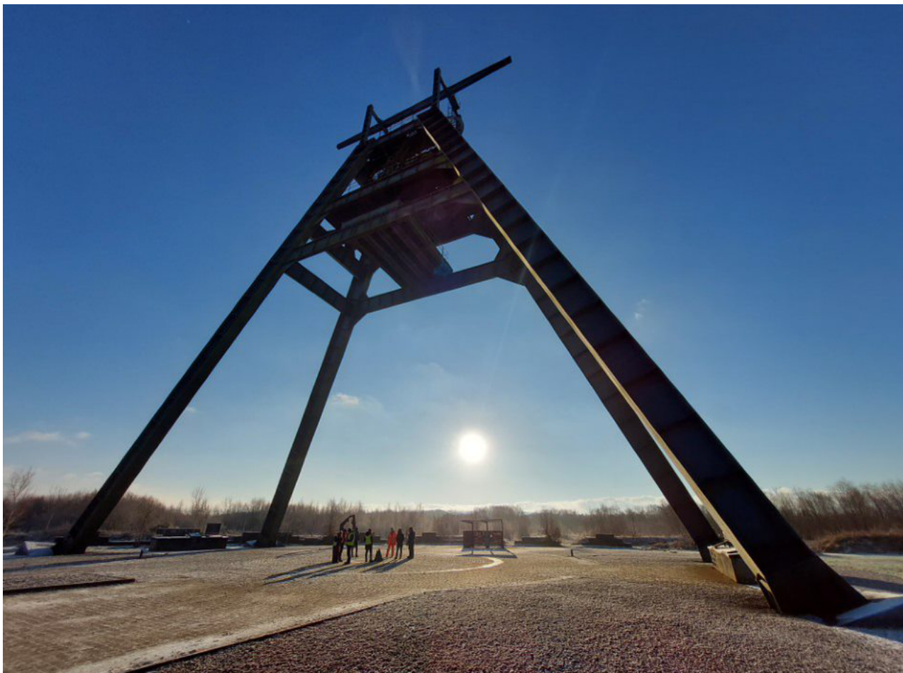
^ Barony A-Frame at Barony Colliery, Scotland. Photo courtesy of Dr Neil Burnside, University of Strathclyde
