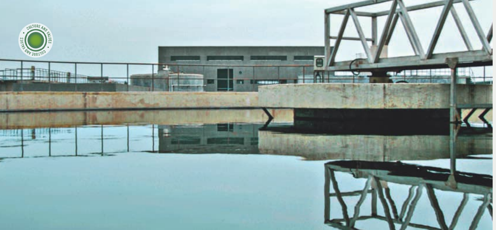
ECCO operates waste water treatment plants at all our tanneries.
