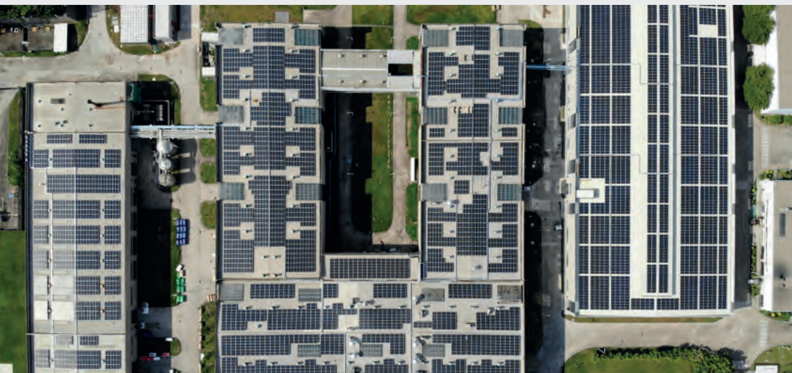
Solar panels on ECCO's new cutting plant and tannery in Xiamen, China
