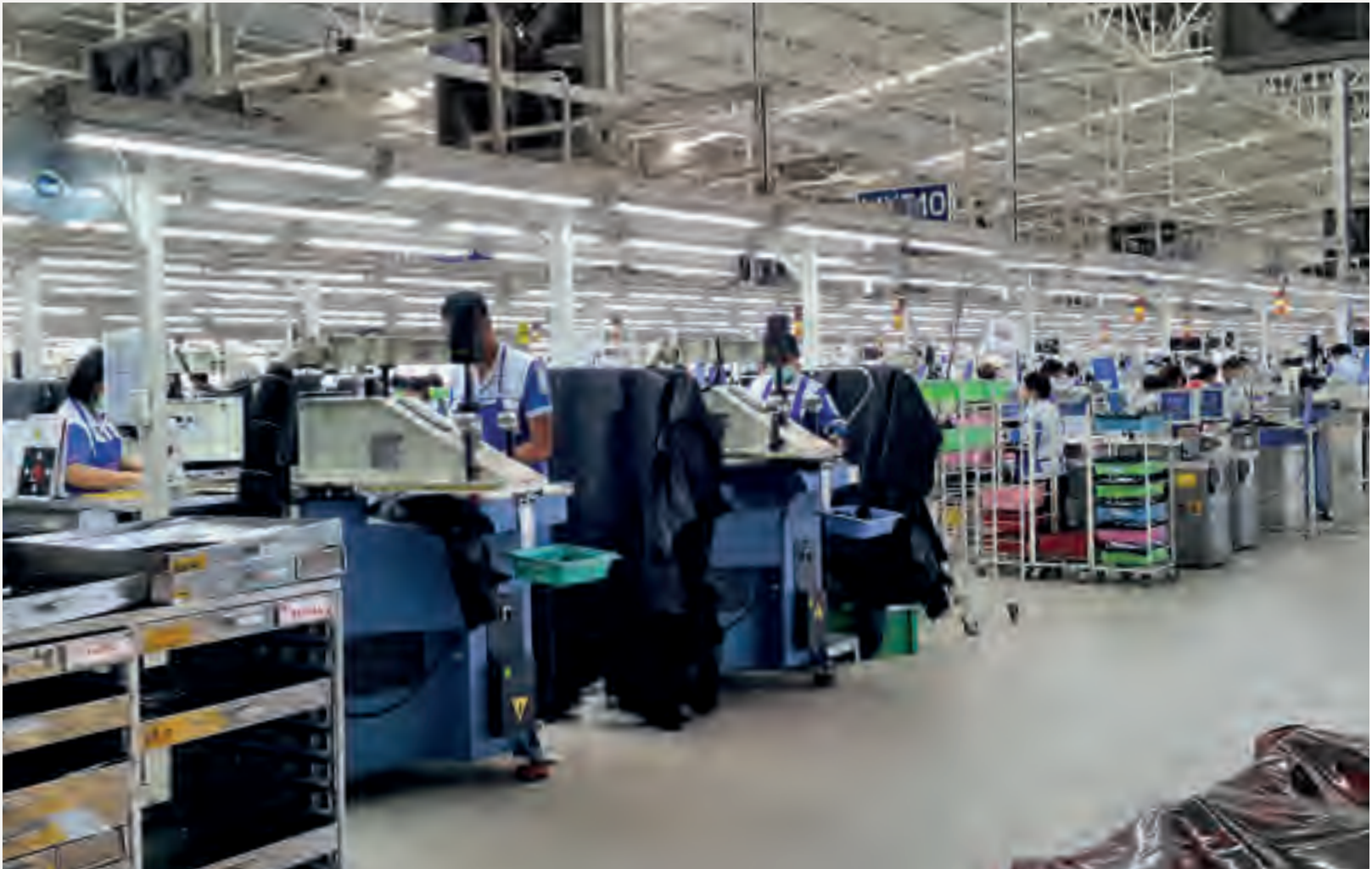
LED lighting has been installed in several of ECCO's factories.
