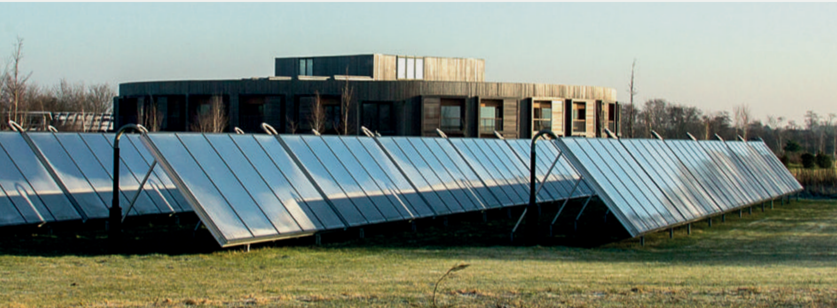
Solar panels at the ECCO Conference Centre in Tønder, Denmark.
