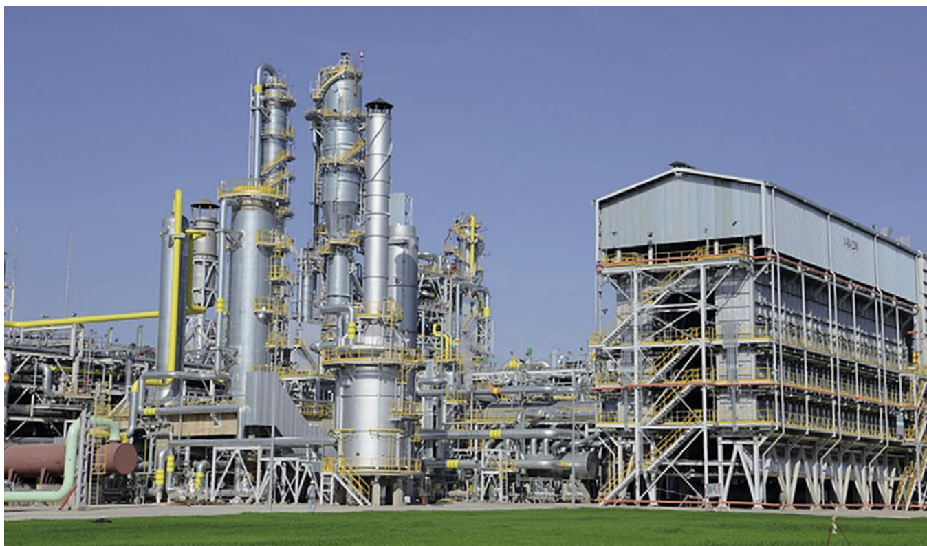
JSC Ammoni can produce only ammonia or both ammonia and methanol in their co-production plant in Tatarstan.
