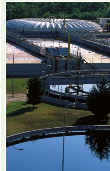
Sludge Treatment Plant Italy
