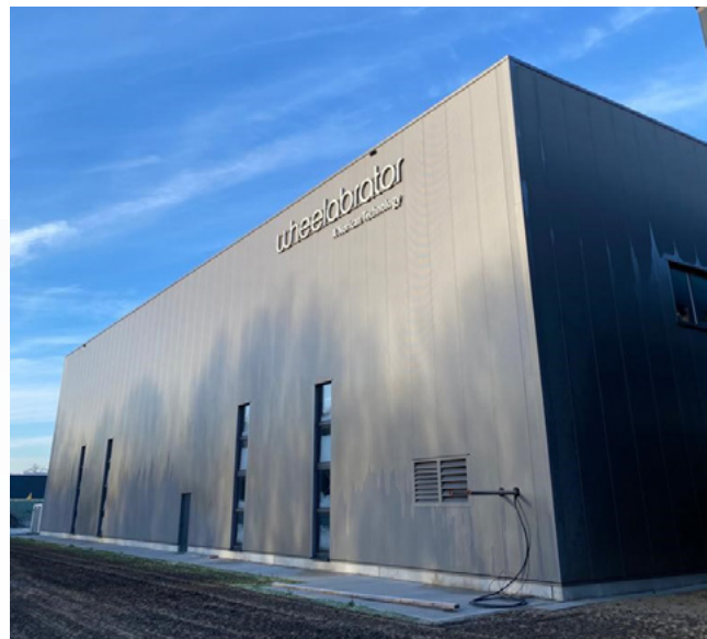
Above: Metelen, Germany
