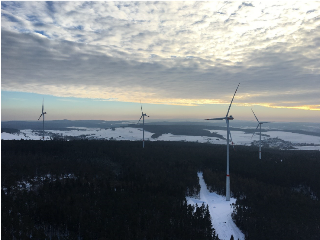
Vindpark Elbenrod, Tyskland. 8xV126 3,3 MW. Idriftsat vinter 2016. Wind park Elbenrod, Germany. 8xV126 3.3 MW. Commissioned in winter 2016.
