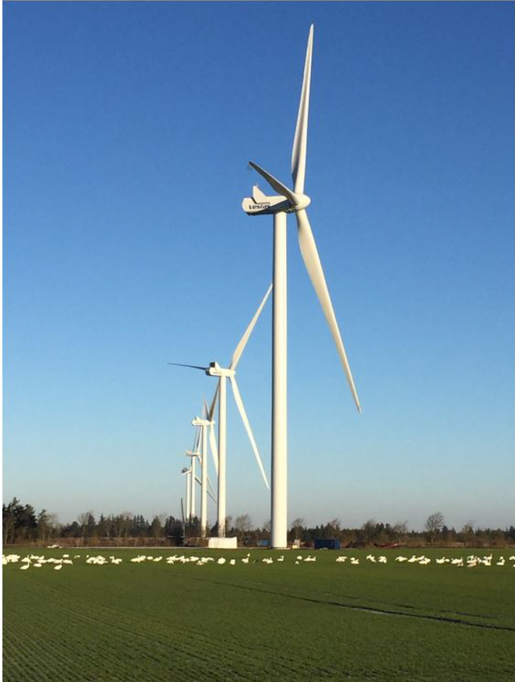
Vindpark Grønkær, Danmark. 5xV126 3,6 MW. Idriftsat primo 2018. Wind park Grønkær, Denmark. 5xV126 3.6 MW. Commissioned at the beginning of 2018
