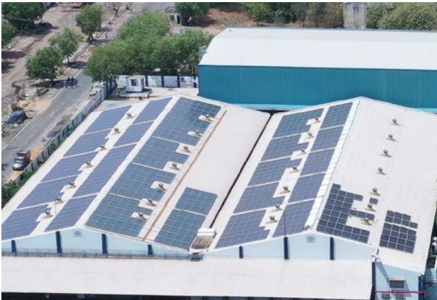
Since 2018 we have systematically been installing solar panels on our warehouse roofs in Missionpharma Logistics India. With the present capacity of 400 kW, we expect solar energy to cover close to 60% of the total energy needs to run our Indian warehouse operations in next financial year.
