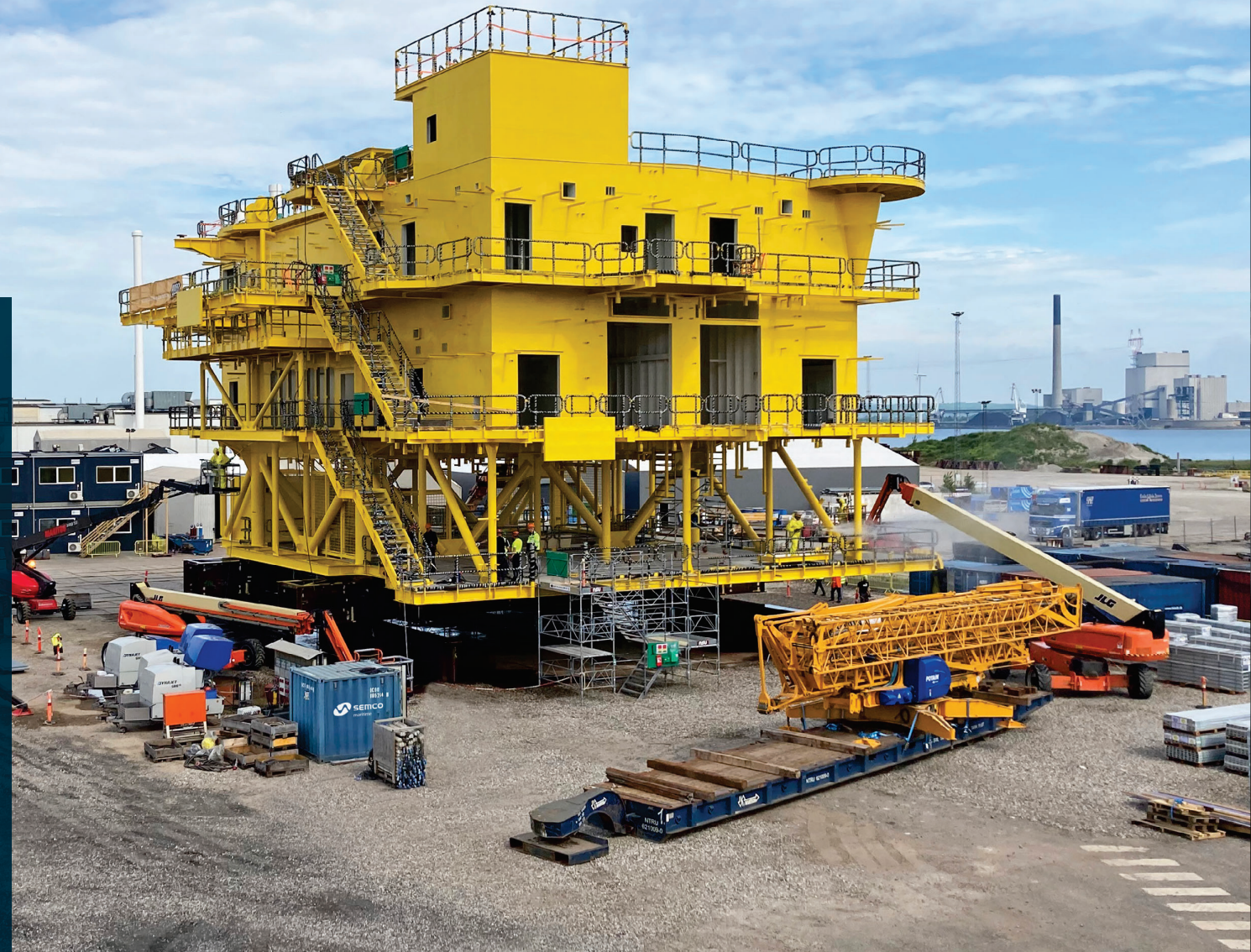
Kaskasi II during installation.
